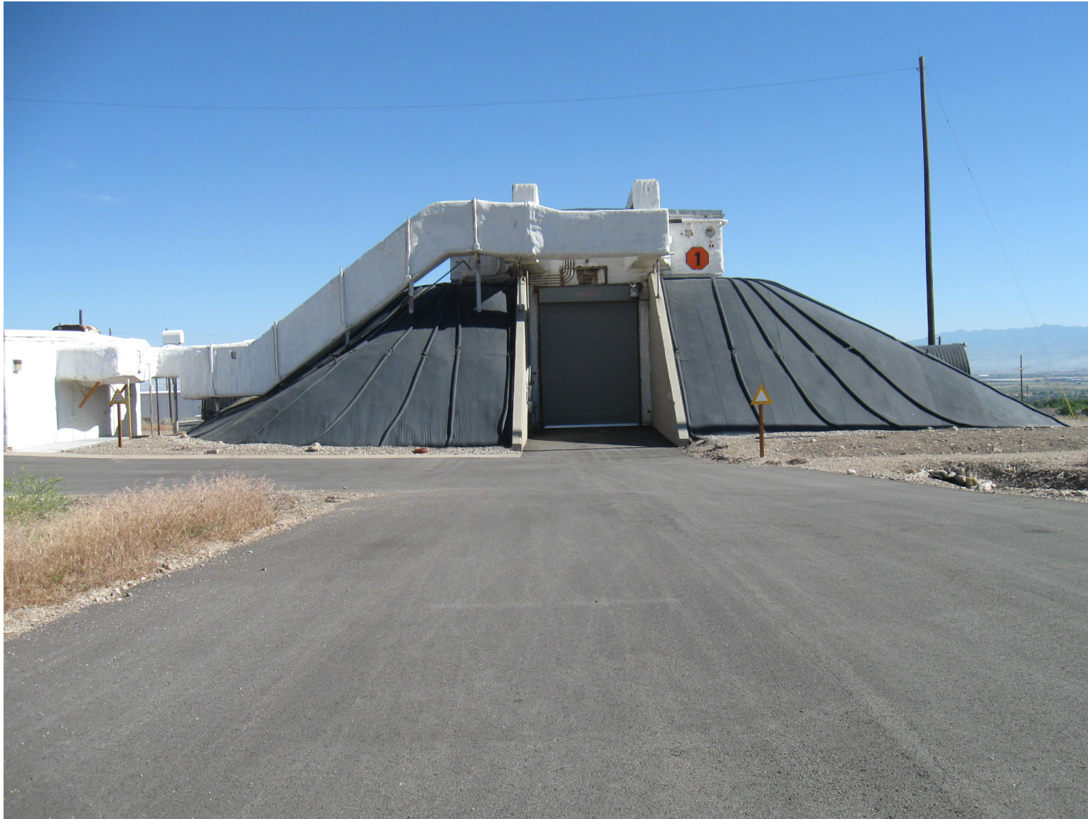
Figure 2-2.10 ES-3 Explosive Storage Building
