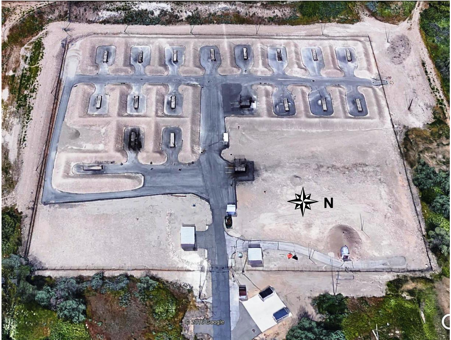
Figure 2-2.4 NIROP BURNING GROUNDS
